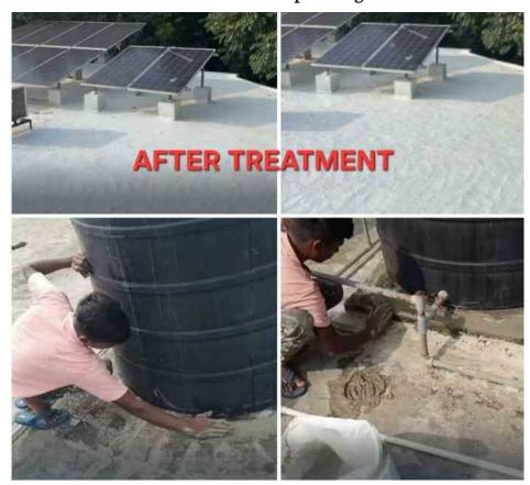
The lobby roof which was leaking profusely at many places was seen and work for waterproofing was allotted to a suitable agency. The roof was thoroughly cleaned, junk material removed and water proofing was done efficiently.
